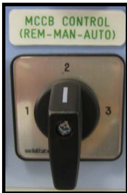
Figure 25. MCCB Control selector switch (-S6)
